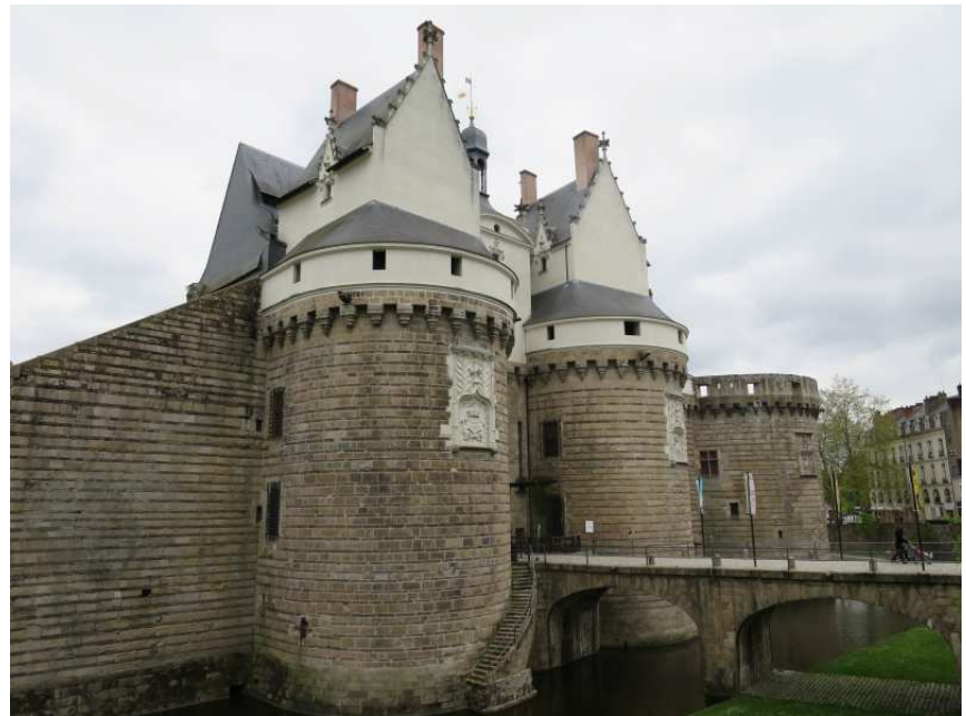
That's massive: Nantes, Fosse du Chateau (during p2k16)
